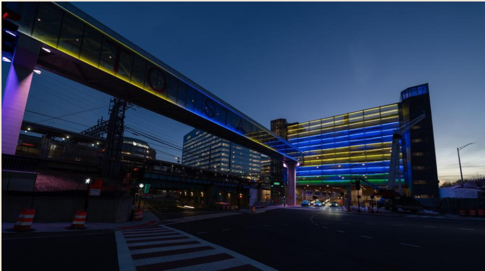
The new Stamford Transportation Center garage and pedestrian bridge
